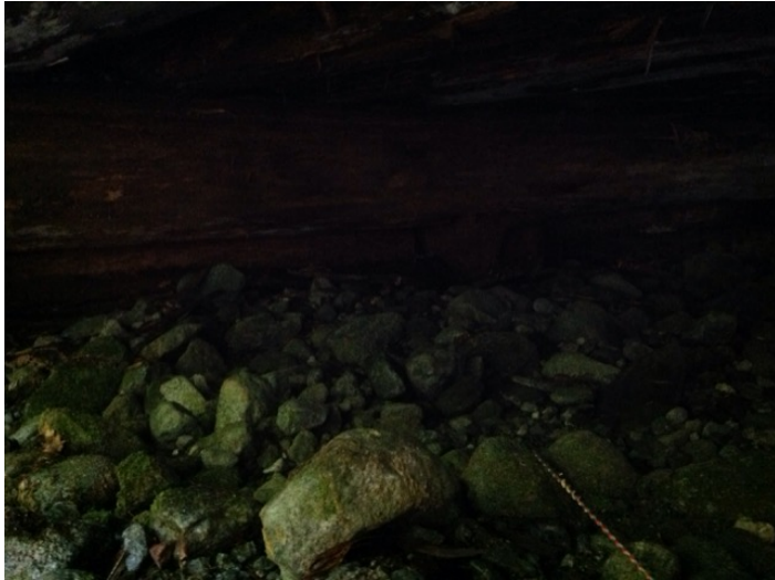
Left Bank Abutment when facing downstream
